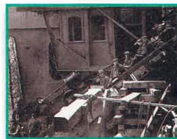
Workers constructing the Cambria Incline
